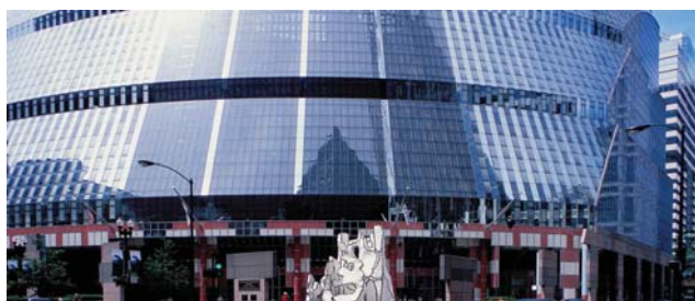
1A1-JH-SC-A2 / State of Illinois Center, Chicago, by H. Jahn
