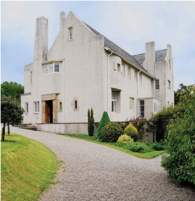
1A1-MCR-HH-1-B7 / Hill House – approach from west
