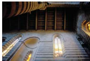
1A2-I-O-D-7-A10 / Nave & Transept
