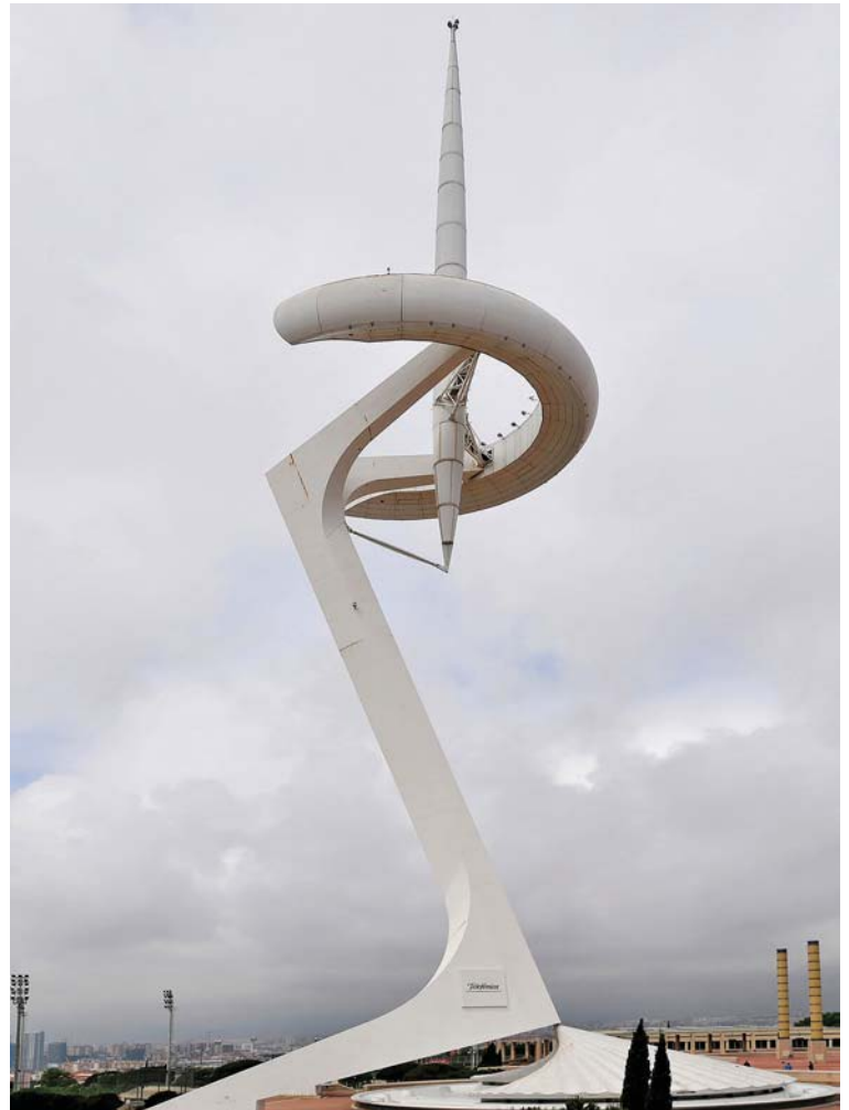
1A1-CS-MCT-A4 / Montjuic Communications Tower
