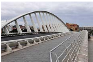
1A1-CS-AB-A5 / Alameda Bridge
