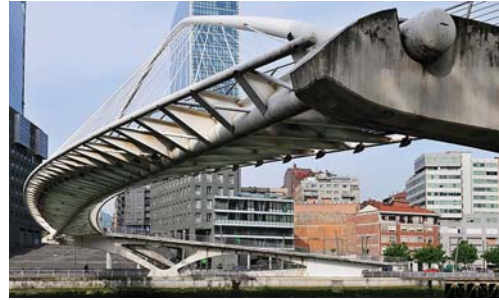
1A1-CS-CVF-A5 / Campo Volantin Footbridge
