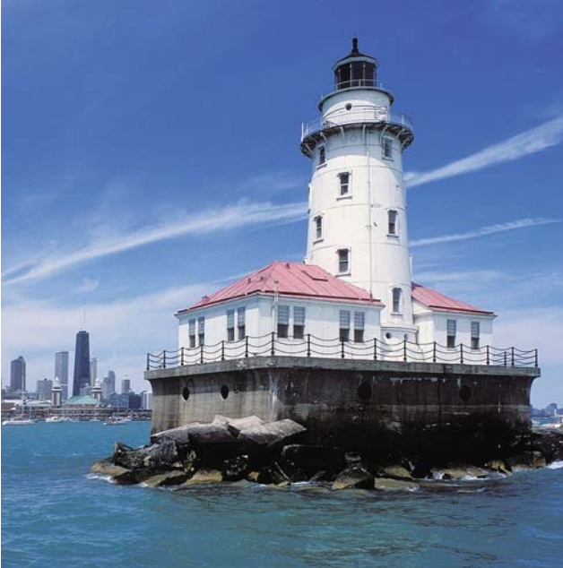
1A2-US-CH-CHL-A4 / Chicago Harbor Lighthouse
