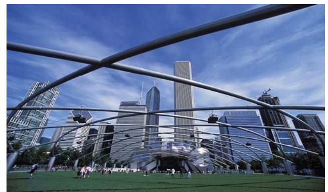
2A2-US-CH-MP-1-F3 / Millennium Park: Jay Pritzker Pavilion
